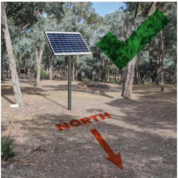
The panel must be positioned in the open and away from shadows and any obstructions.
